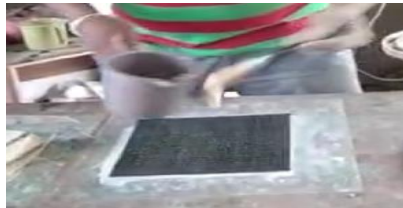
Figure 12 Place the first layer carbon fiber
