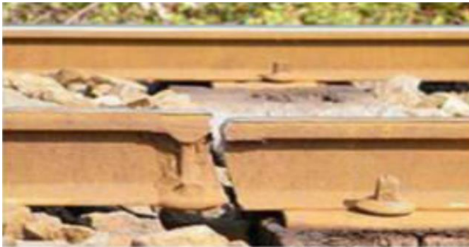
Figure 2. Railway Track Crack
