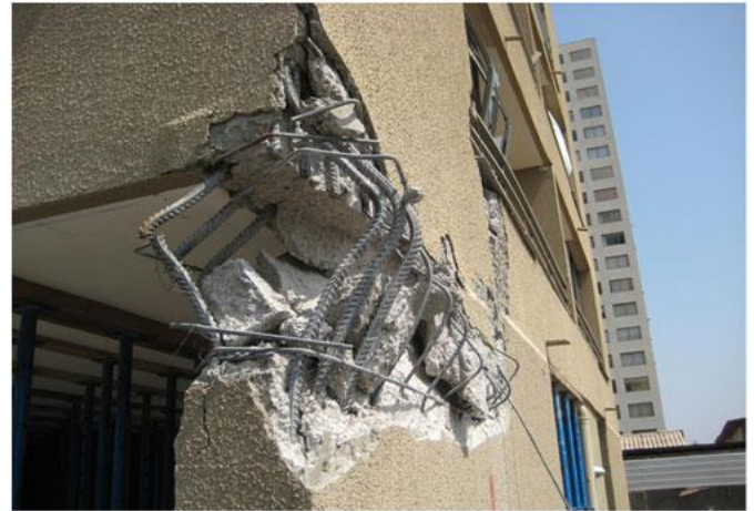
Fig.2 Column failure (absence of tiers, buckling of longitudinal bars)
