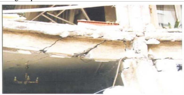
Fig.1 Diagonal cracks of the beam and failure at the column top
