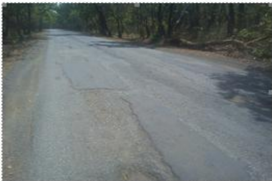
Figure 2 Rough road condition
