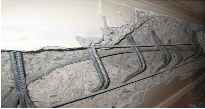
Figure No 2: Concrete Crushing And Buckling Of Longitudinal Reinforcement Initiating At Wall Boundaries And Propagating Along The Length Of Wall Segments
