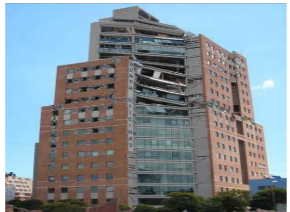
Figure No 5: Concentrated Damage At: (A) Wall Discontinuities; And (B) Structural Irregularities
