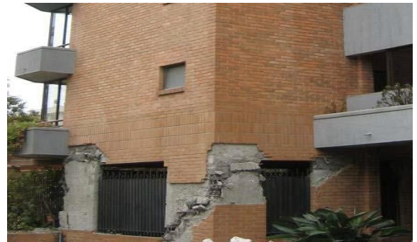
Figure No 4: Overall Wall Buckling Behavior
