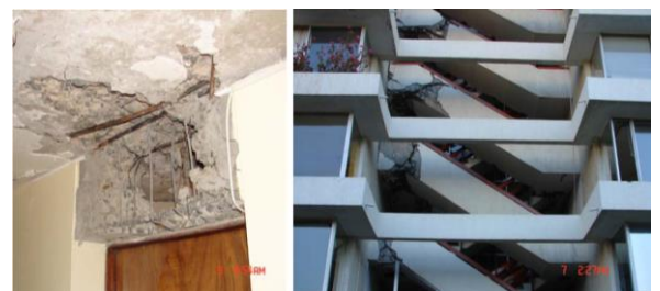
Figure No 6: Concentrated Damage At: (A) Coupling Beams; And (B) Cast-In-Place Concrete Stair Elements Description of Observed Damage to Wall Boundary Elements
