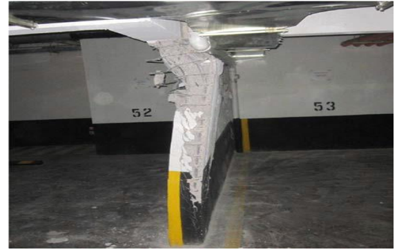
Figure No 4: Overall Wall Buckling Behavior
