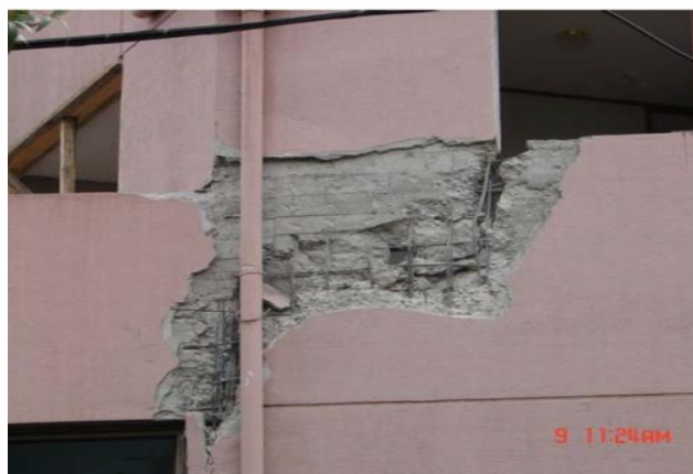
Figure No 3: Shear Failures In Vertical And Horizontal Wall Segments
